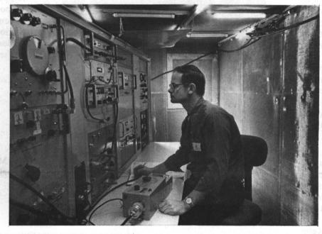
IN SPECIAL SCREEN ROOM of the microwave measurements laboratory, Bob Moyer makes attenuation measurements. The area is screened completely from random RF noise.
